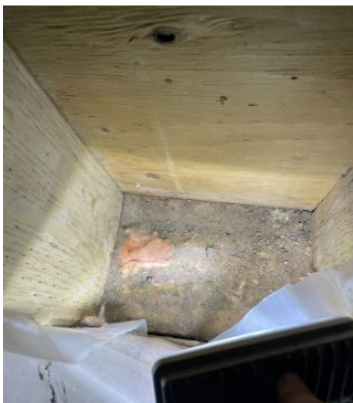
Cavity of stud bay in PWF
