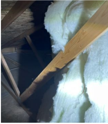
Insulation bundle in garage attic
